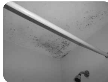
Normal condensation related mold growth easily cleanable by the tenant or property manager.
