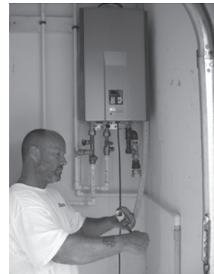
Rinnai Tankless Hot Water Heater Install
